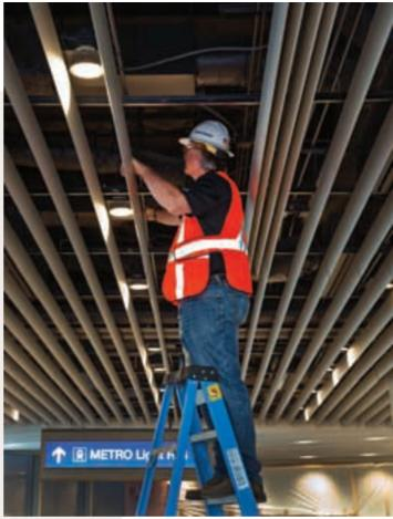
The High Profile Series creates a clean plenum mask that offers easy point access to lighting, HVAC, security, audio and fire safety systems. Baffles easily slide or demount to allow hassle free access for maintenance. The spacious appearance is ideal for large interior spaces, when a more open ceiling plane is desired.
